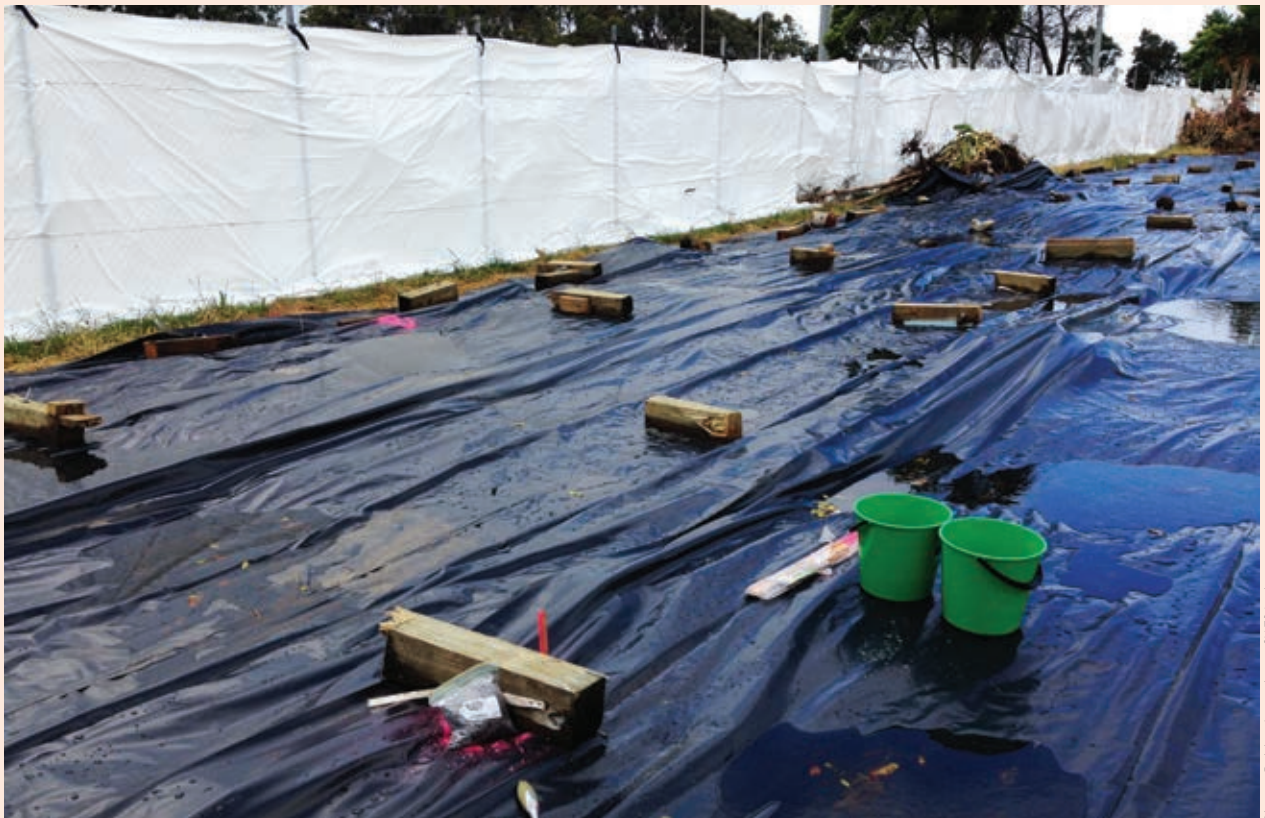
Figure 27. Temporary cover of contaminated soil.
